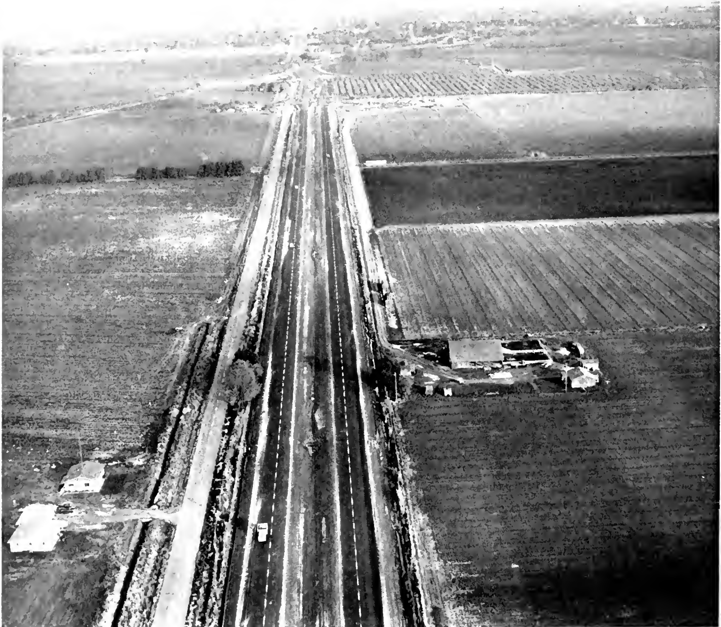
This aerial of Allamant Pass Tracy Freeway is looking east toward Tracy
